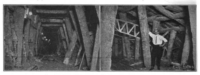
FIG. 11. UPPER HEADING AND ENLARGEMENT; MAIN TUNNEL
