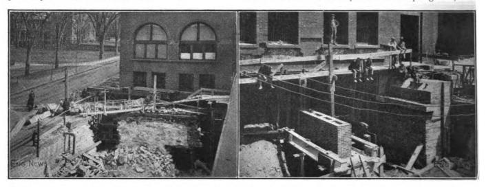
FIG. 7. BEGINNING NEW FOUNDATIONS, DRAINAGE DRIFT FIG. 8. STEELWORK UNDER WEST WALL AND FOUNDA-AT THE RIGHT TIONS OF DRIVEWAY ARCH
