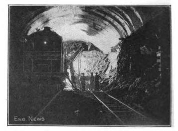
FIG. 12. REMOVING BENCH WITH SHOVEL; EAST SIDE TUNNEL, PROVIDENCE
